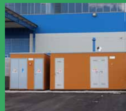
PREFABRICATED MV/LV CONCRETE COMPACT SUBSTATION
